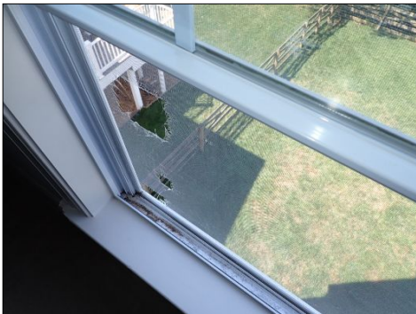
Damaged Screens
