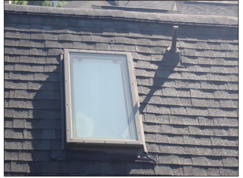
Skylight & Vent Pipe
